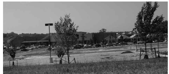
Acme-Lowe's shopping center on Route 41, London Grove
