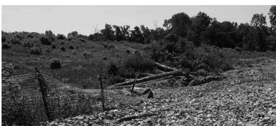
Construction, Line road, New Garden
