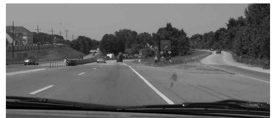
East Marlborough and Kennett Township at the beginning of the limited access highway
